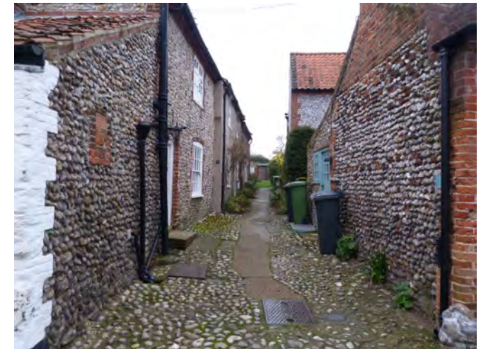
Informal flint cobbles, paving and planting on a lobe off the High Street
