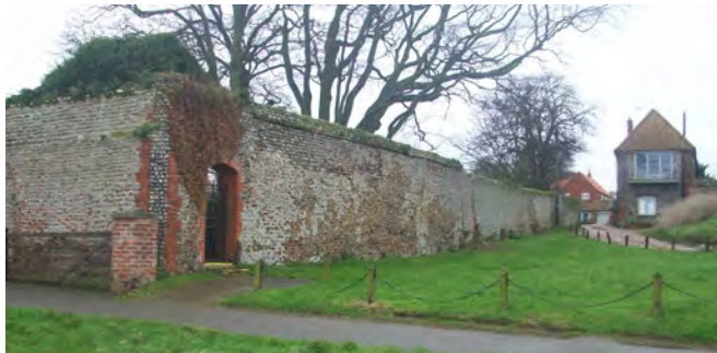
High walling (Grade II listed) enclosing Manor Hotel
