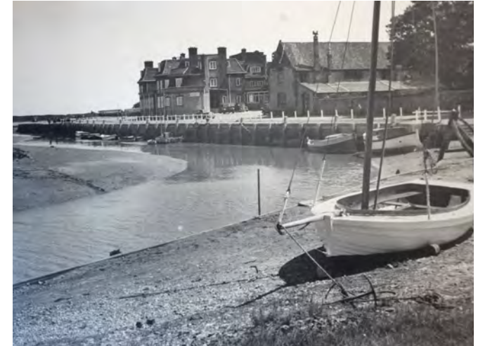
Blakeney Quay, post-1935 (Image courtesy of Norfolk Heritage Centre, Norfolk and Norwich Millennium Library: Blakeney)
