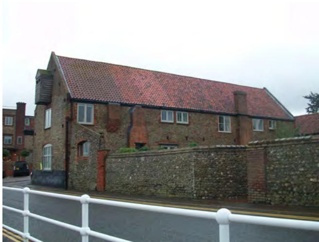
Two and a half storey barn conversion along the Quay
