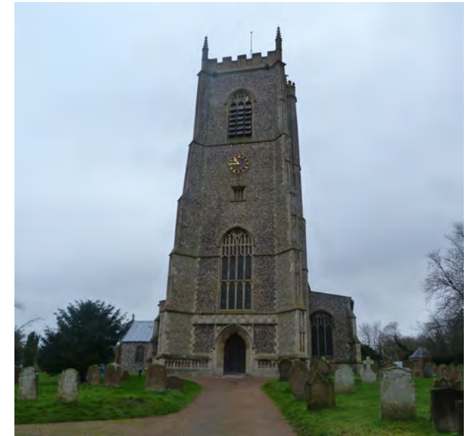
Blakeney Parish Church
