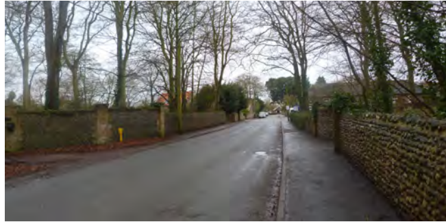
Walls flanking Wiveton Road on both sides
