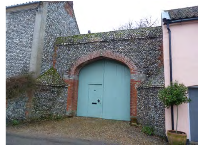
Gateway and wall on High Street, with sloped flint capping detail
