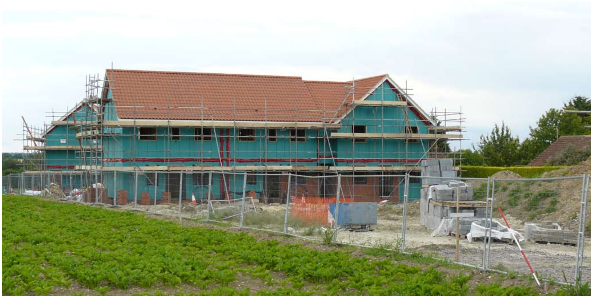
New social housing at Langham under construction
