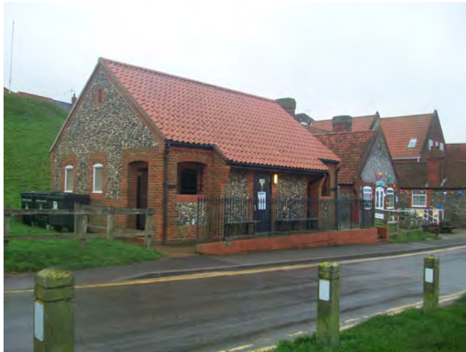
Ad-hoc railings outside the public toilet, Mariner's Hill and village hall
