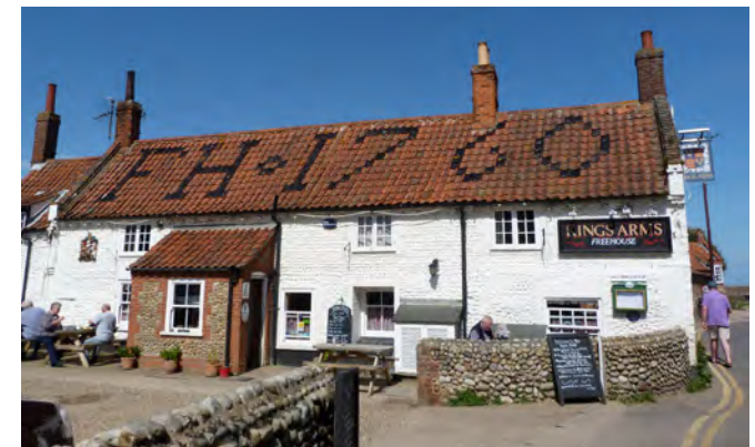
The Kings Arms with decorative roof tiling
