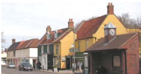
Figure 33 : Attractive houses on the east side of White Lion Street
