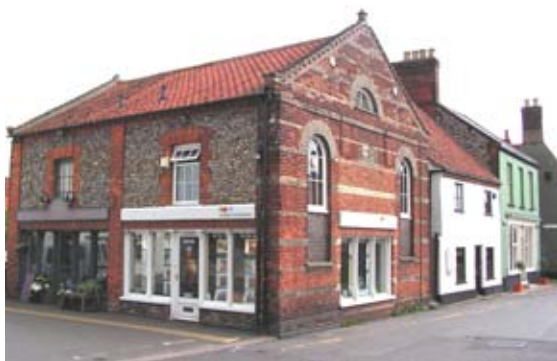
Figure 24 : Chapel at the corner of Chapel Yard and Albert St.
