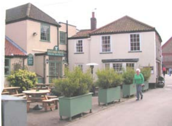
Figure 47 : Feathers Yard, looking towards Budgen's car park
