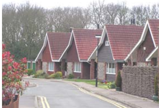
Figure 41 : Houses of Town Close
