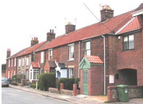
Figure 36 : Houses at the end of the Conservation Area on the east side.
