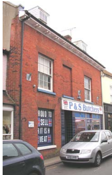
Figure 21 : Early house with a 20th century shop front, Bull St.
