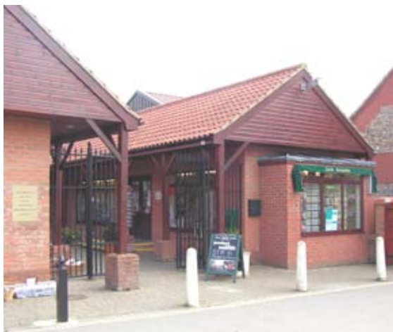
Figure 48 : Unattractive shops on the east side of Feathers Yard
