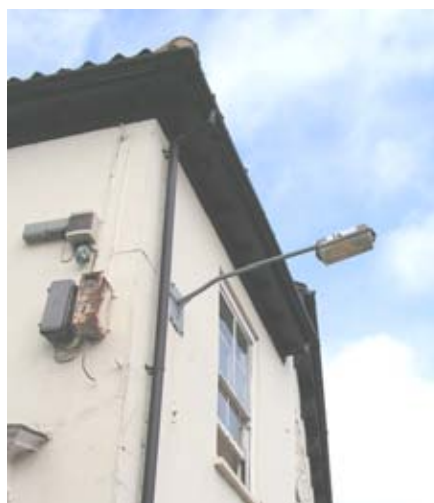
Figure 70 : Lamp attached to the side of a building in Bull Street
