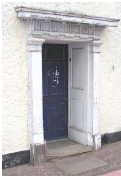
Figure 64 Doorcase of a listed building in need of maintenance on the Norwich Road.
