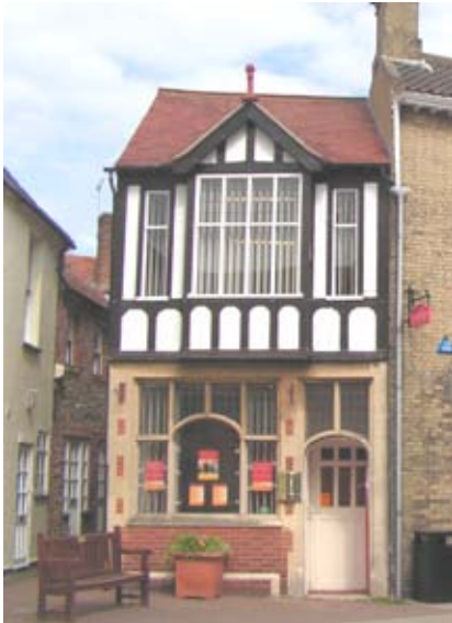
Figure 61 A former late Victorian bank in Market Place
