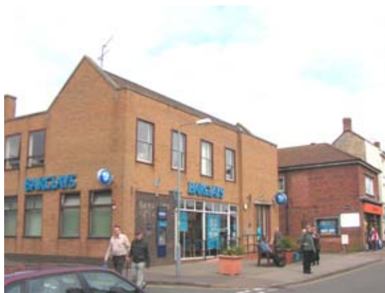
Figure 14 : Barclays Bank and forecourt with town sign.
