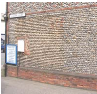
Figure 56 Early brick and cobble walls at the entrance to Baker's Yard
