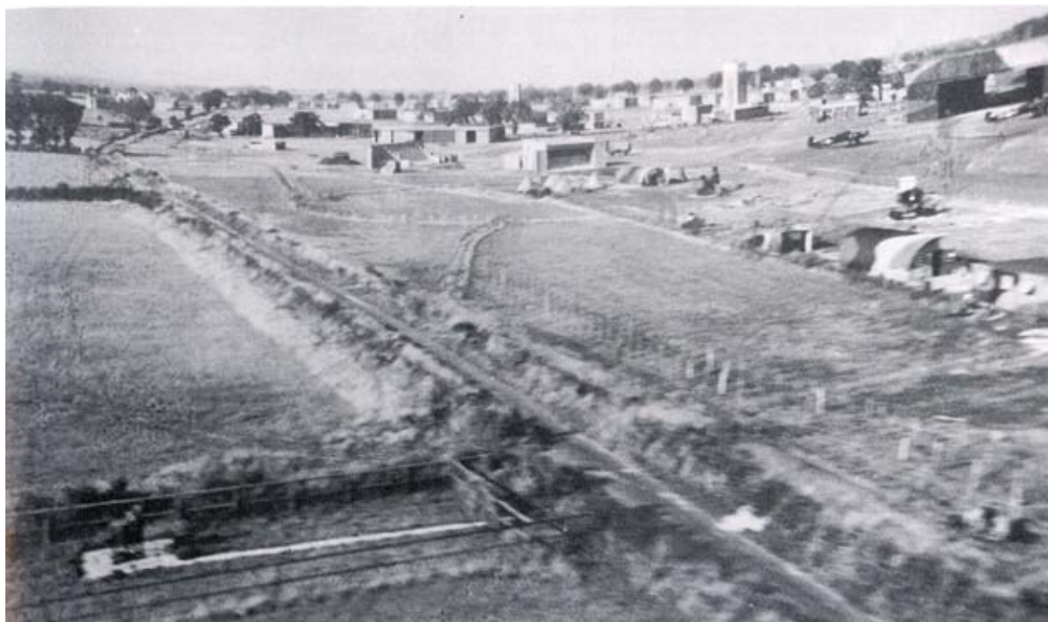
Low Level view of the base in the 1940s showing early development. In the distance the Water Tower proposed for Local Listing is clearly visible.
