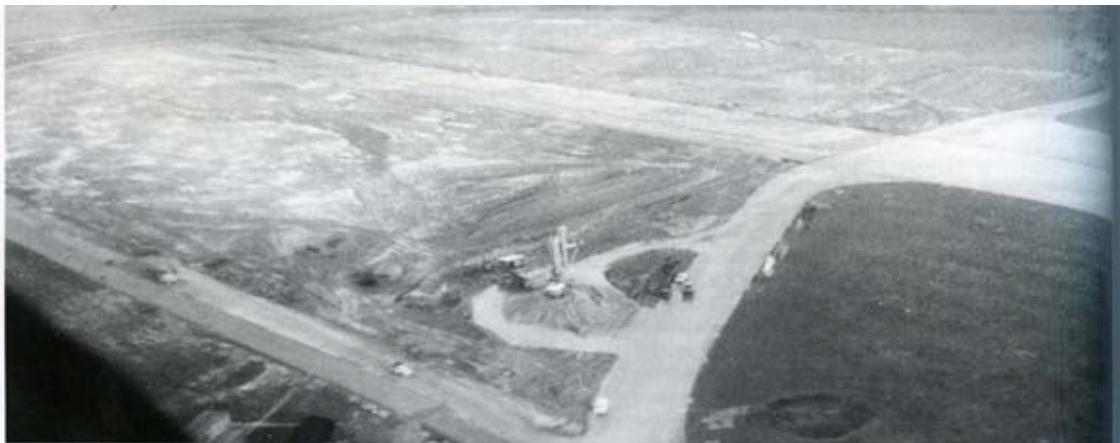
The runway extensions under construction 1957
