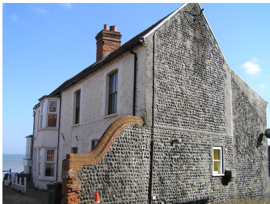
Figure 34 : A good example of coursed flint work within the Conservation Area
