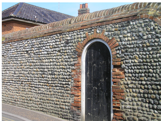
Figure 30 : One of the many arched door openings in high flint walls.
