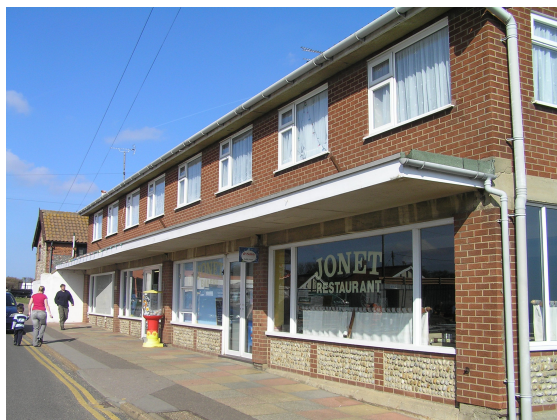
Figure 41 : The 1960s commercial development on Beach Road
