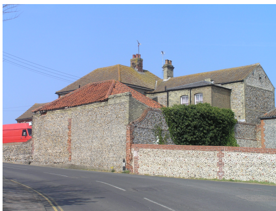
Figure 35 : Another example of coursed flint within the Conservation Area
